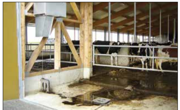
▲ Mounting drive winch EW4 and guide pulley
