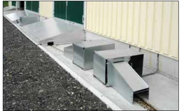
▲ Drive winches EW4 and cross canal covering
