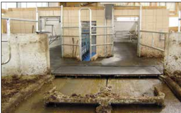
▲ Foldable cross channel cover in front of the milking parlour
